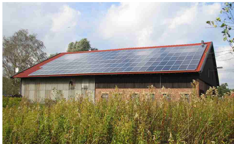
Photovoltaikanlage 27 kWp in Waltrop (Solarmodule BP 7175)
